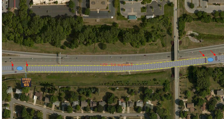
Figure 6.4 The Test Segment of I-235 from Valley West Dr (NB) to exit 2 in Des Moines, IA. Arrows indicate location of volume sensors. Elliptical regions imply the entry or exit location for on-ramp or off-ramp vehicles. Dynamic speed limit sign is at the left vertex of the segment.
